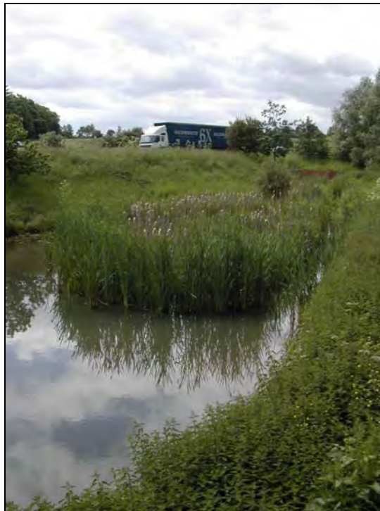
Figure 2 – Typical example of a highway drainage balancing pond
