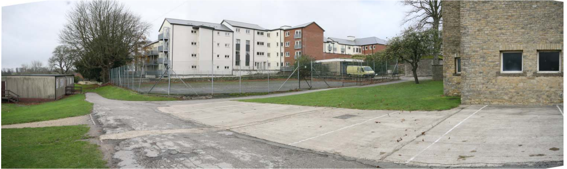
PH04 - EXISTING PARKING AND TENNIS COURT
