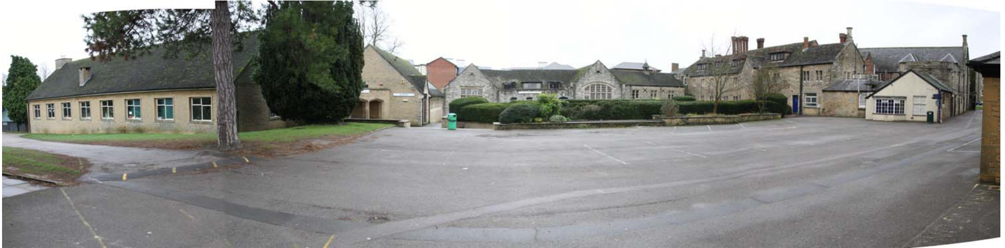
PH02 - EXISTING CAR PARK 01 - 13 Spaces
