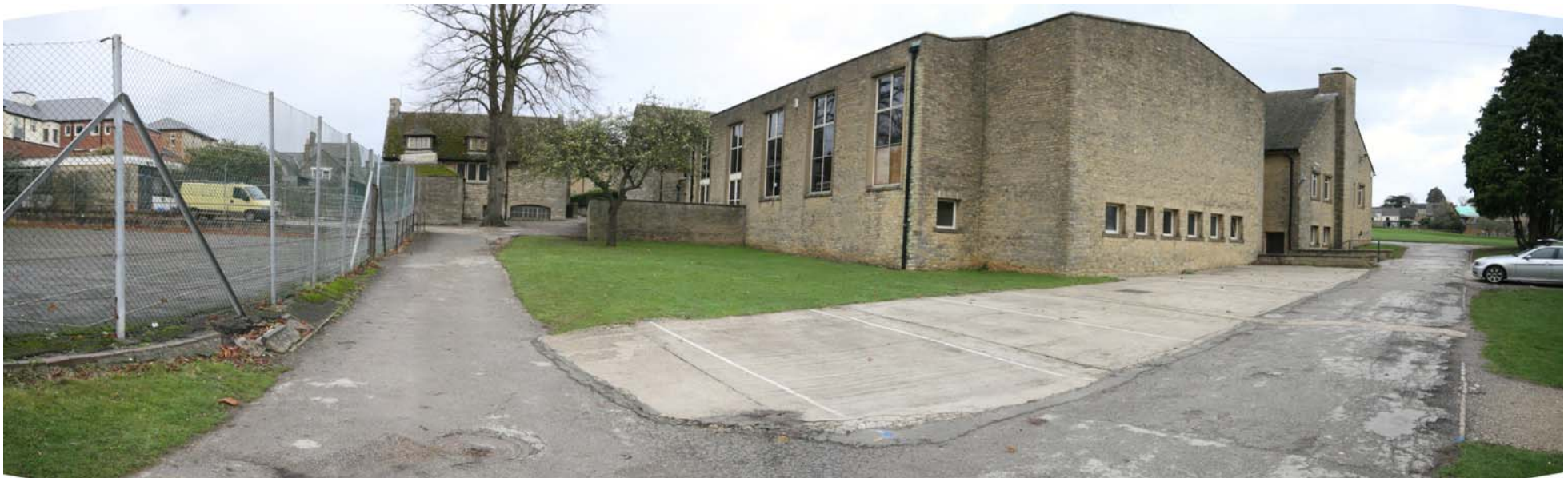
PH03 - EXISTING CAR PARK 02 - 8 Spaces
