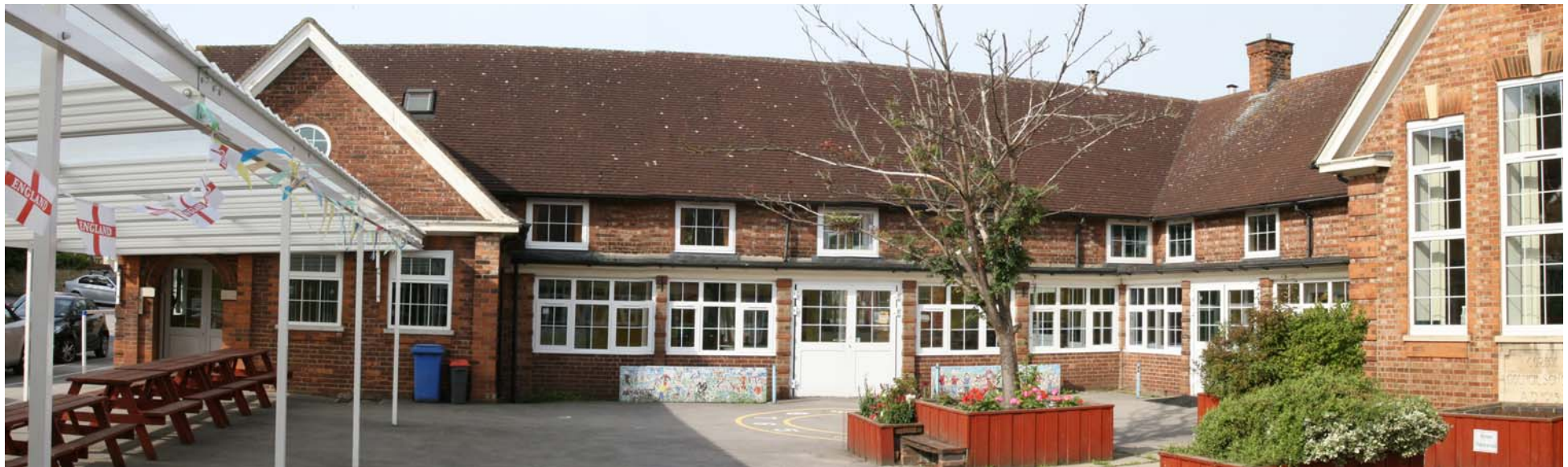
Photo 02 - Existing East Elevation - Inner Courtyard
