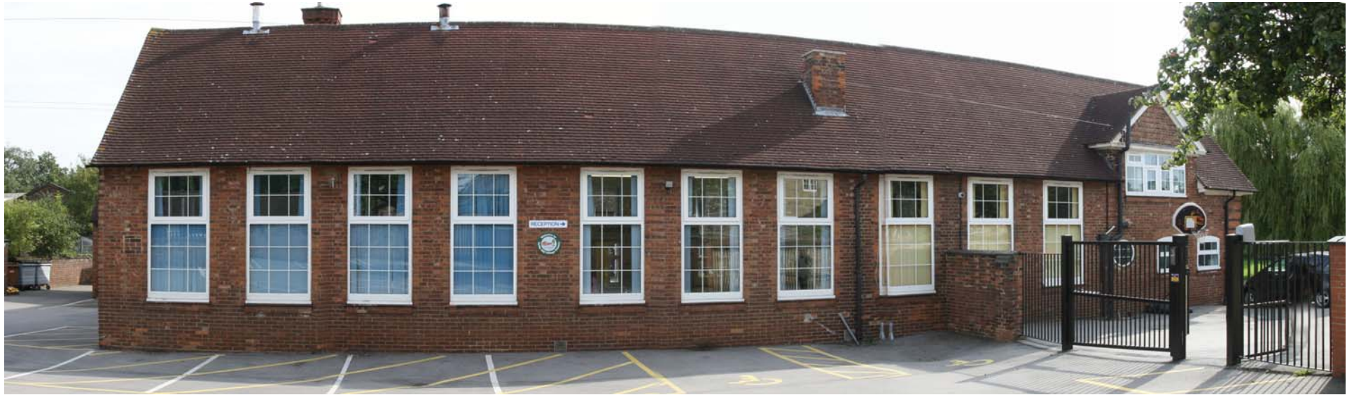
Photo 04 - Existing West Elevation - Staff Car Park Entrance
