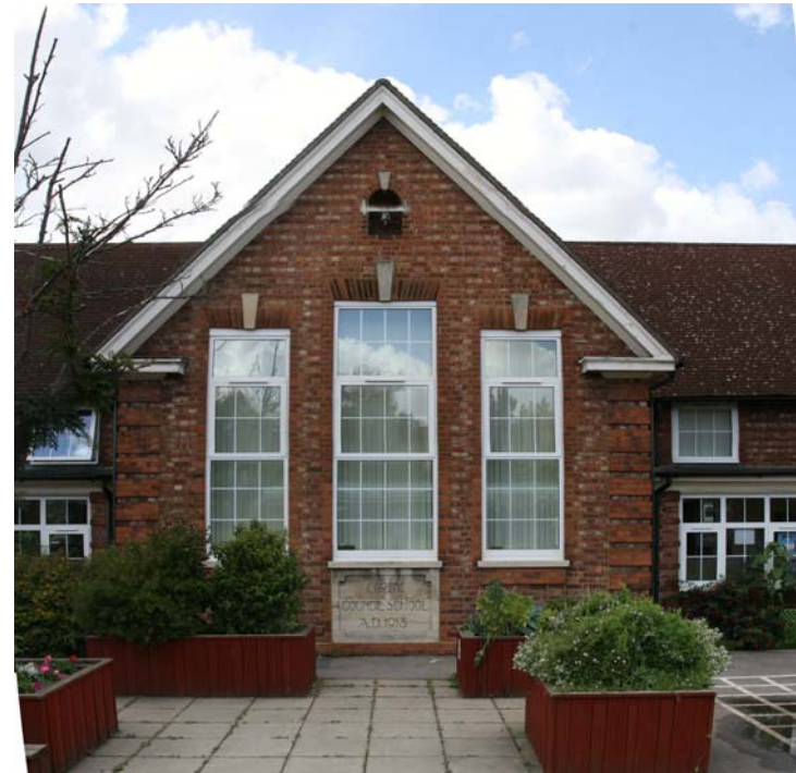
Photo 06 - Existing Rear Gable to Hall and Building Plaque
