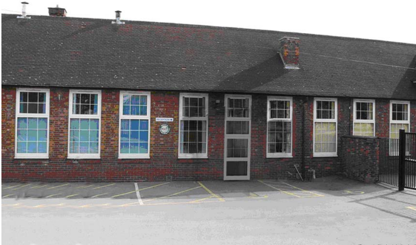
Photo 10 - New Reception Access
