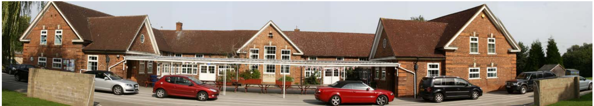
Photo 01 - Existing South Elevation
