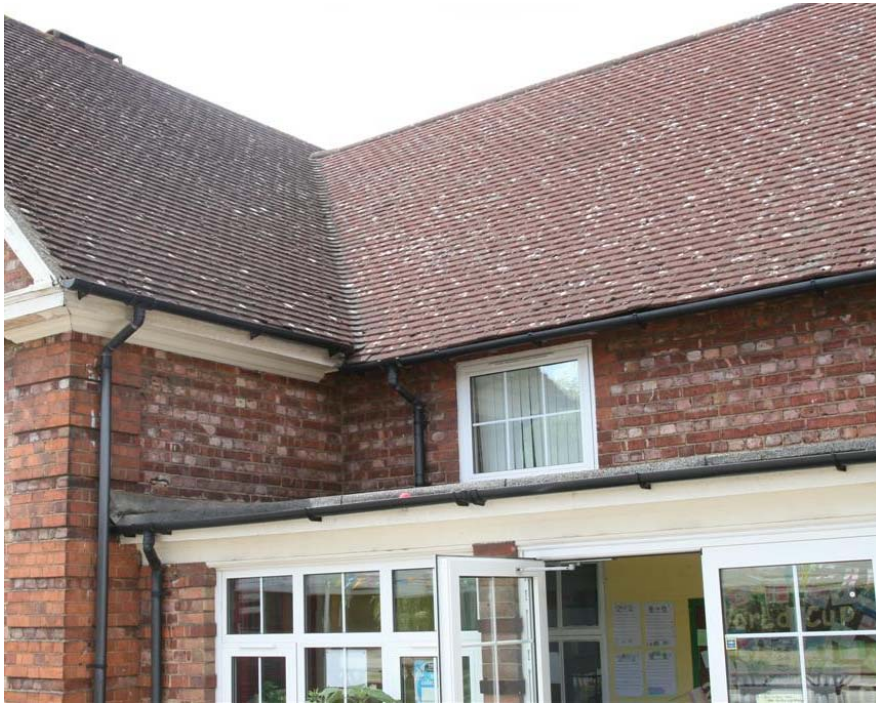
Photo 05 - Existing Soffit Details
