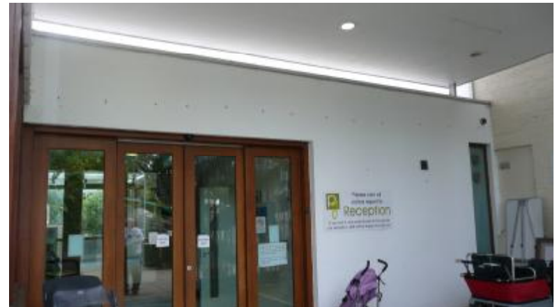
VIEW TO LIFT POSITION
