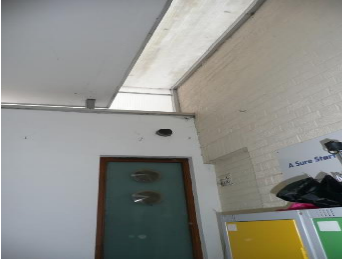
VIEW TO LIFT POSITION
